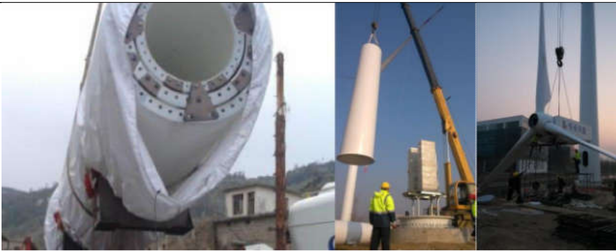
Fig.5 transportation of tower sleeve and installation of tower.
